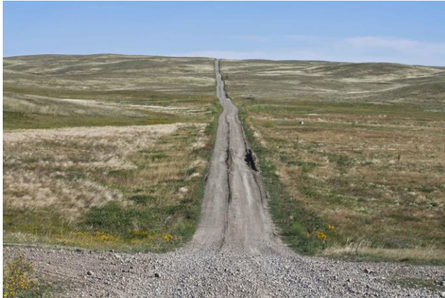
Access road through a low lying area in a dry year.
